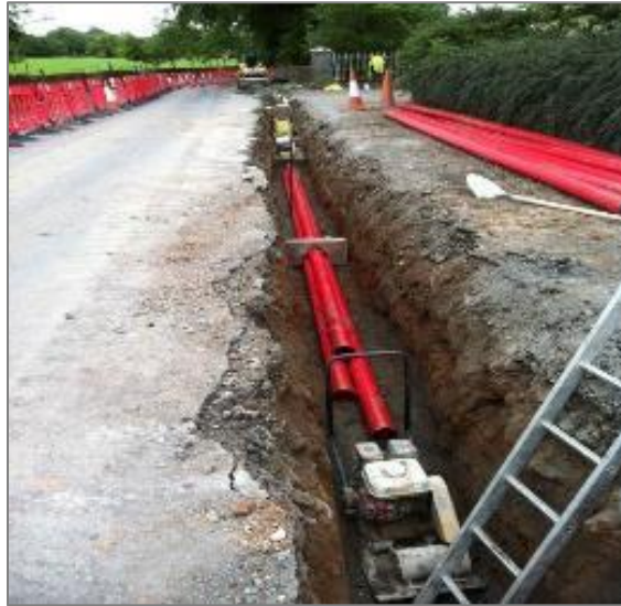
Figure 3 - 110kV Underground Duct Installation
