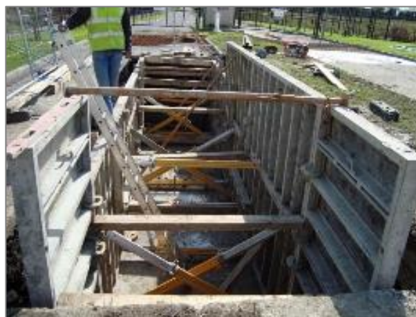
Figure 9 - Typical joint bay under construction (in-situ)
